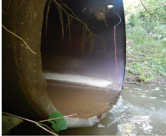
Figure 6. A culvert that has become perched at Hart Creek site 2.
