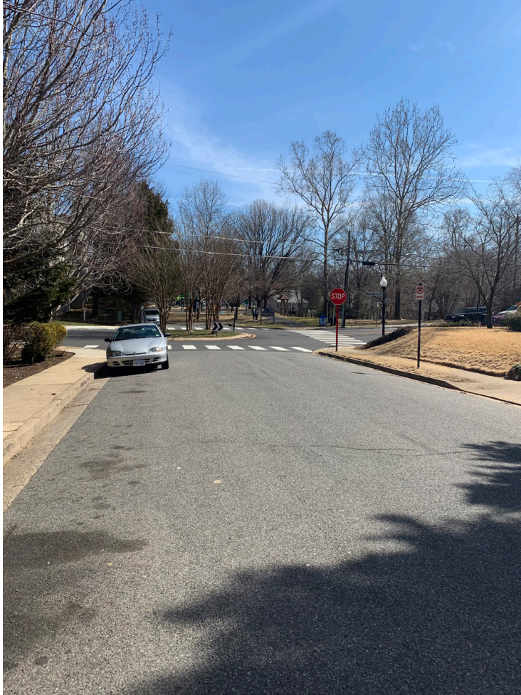
Figure 59 Photo Record Series Existing Conditions - #8 - photo by Author
