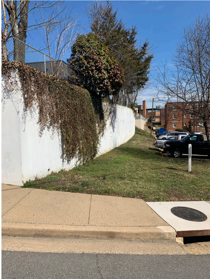
Figure 53 Photo Record Series Existing Conditions - #3 - photo by Author
