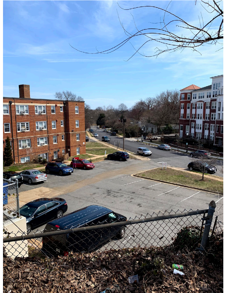
Figure 54 Photo Record Series Existing Conditions - #3a - photo by Author
