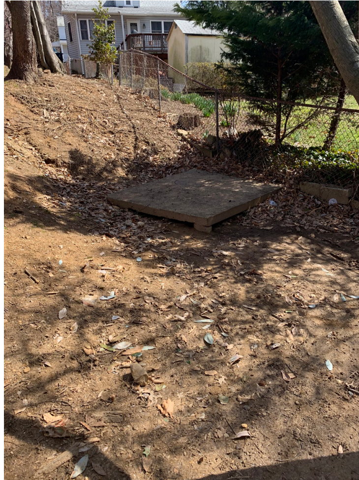
Figure 63 Photo Record Series Existing Conditions - #12 - photo by Author
