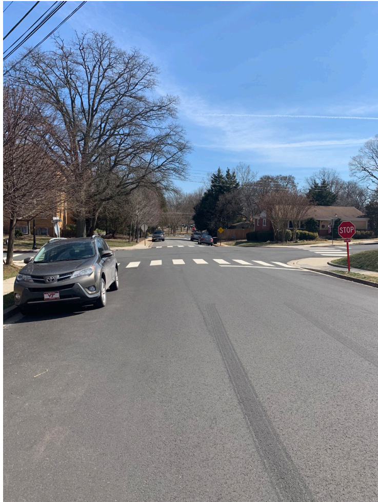
Figure 56 Photo Record Series Existing Conditions - #5 - photo by Author
