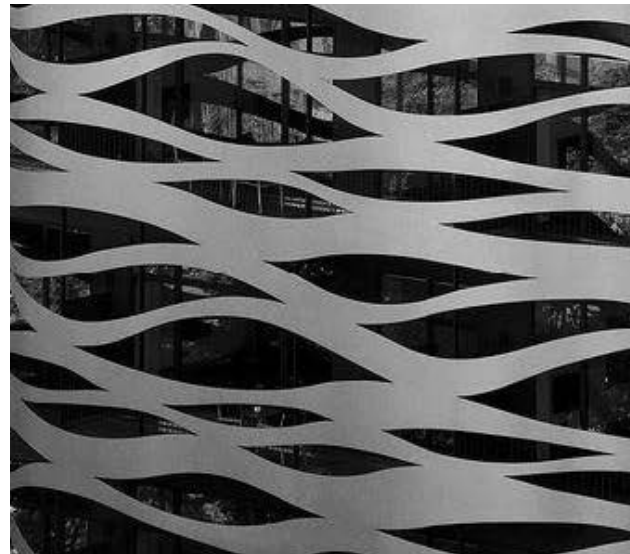
Facade Renovation "Suites Avenue Aparthotel", 2009, Barcelona, Spain. Photographed by Iwan Baan
