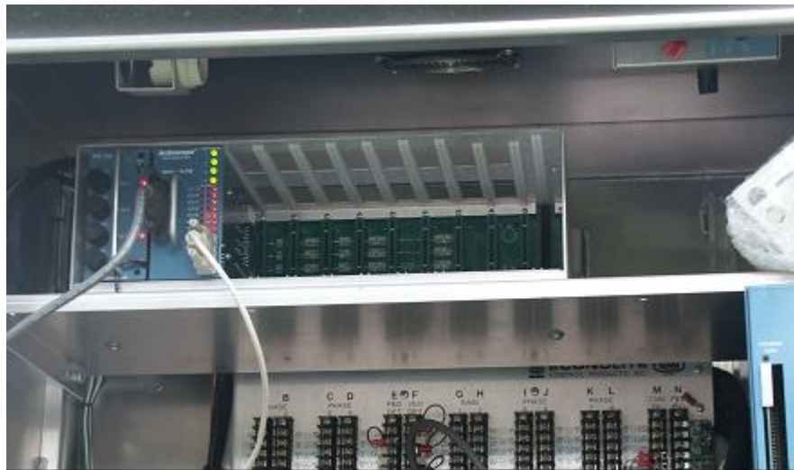
Figure 3.7 - Mini-Hub II in Major Control Panel
