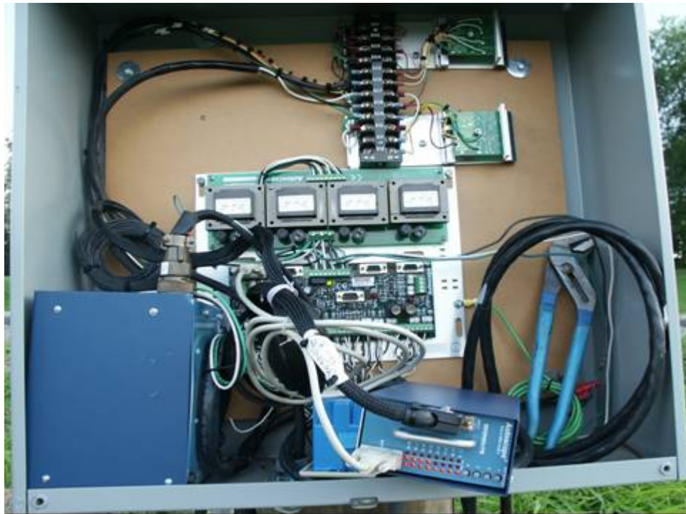
Figure 3.8 - Minor Control Panel
