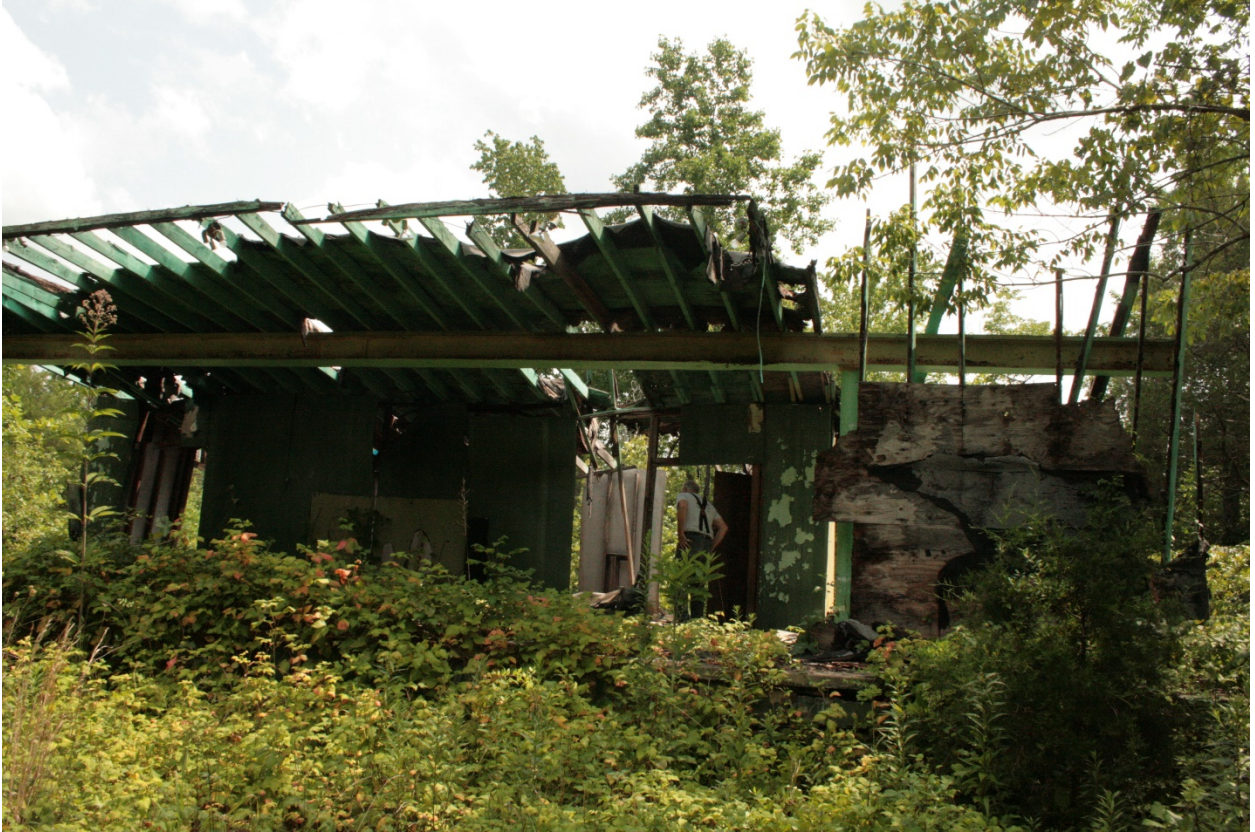
Figure 4. The Camp Springs Festival Stage as it appeared the summer of 2015, overgrown with the roof deteriorating. Robert “Quail” White can be seen walking on the stage. Photo by Jordan Laney. [Used with permission]
