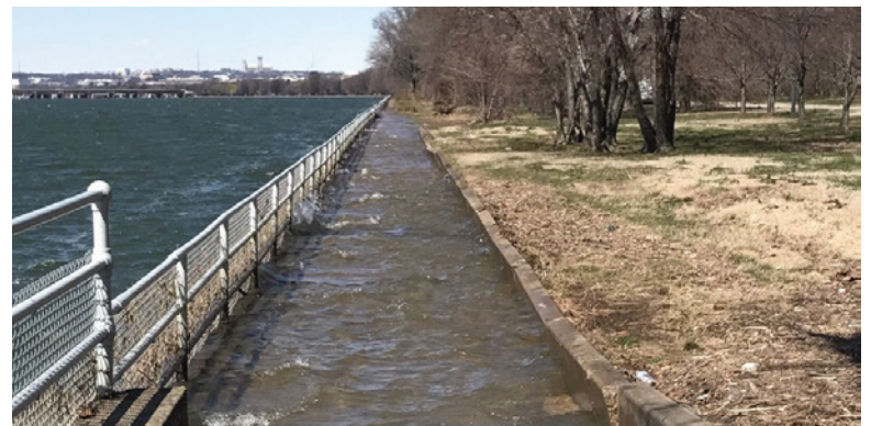
Fig 22-23: Pictures of Hains Point deteriorating edge
