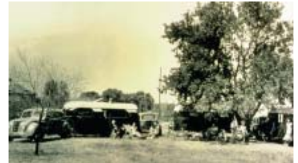
Figure 2.2 Camping along the roadside. (MHI)
