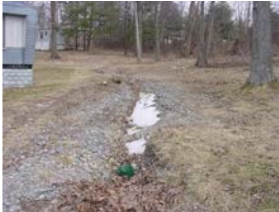
Figure 5.26 Deep rut cut by storm water runoff. (Bean)
