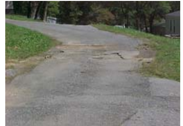
Figure 5.23 Old roads are in need of repair. (Bean)
