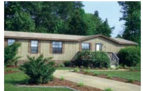
Figure 5.4 Though the landscaping received approval, the uncovered deck at the front entrance did not. (MHI)
