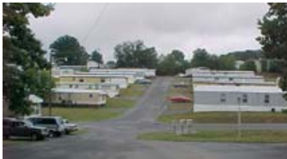
Figure 5.28 Rows of homes marching down a less steep portion of the hillside. (Bean)
