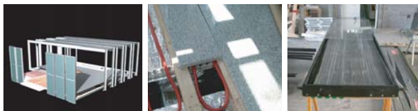
Top: 3d model of the house showing radiant floor. Right: view of the upper east corner showing thermal panels, PV panels, and structure. Bottom left: 3d model showing the thermal south wall and radiant floor. Bottom middle: radiant floor with granite tiles for thermal storage. Bottom right: custom made thermal panels under construction.
