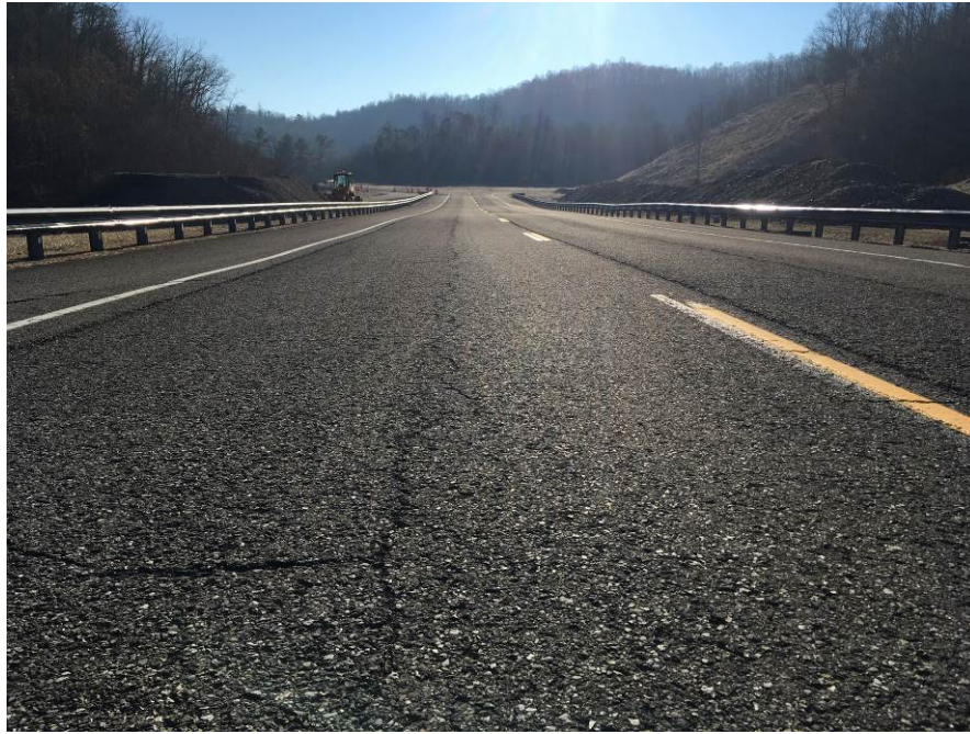
Figure 2. Photo. Smart Road asphalt surface at test site.
