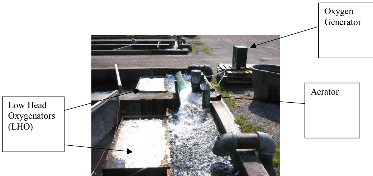
Figure 1. Picture of oxygenated raceways; oxygen is produced by the SeQual generator and then diffused via the LHOs.
