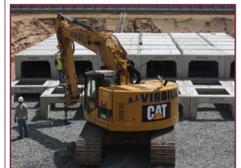
*Concrete Pipe & Precast's new stormwater detention/retention system, Retain-It, optimizes storage while maintaining a small footprint.*
