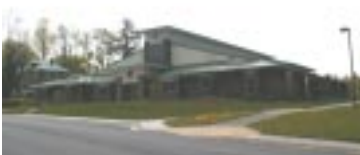
A. Front entrance (closed)
