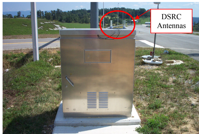
Figure 9: Intersection Cabinet with DSRC antennas
