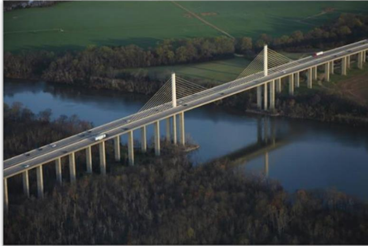
Figure 1.1: Aerial View of Varina-Enon Bridge
