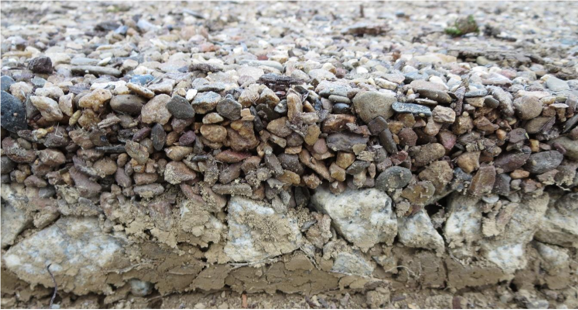
Figure 4.2. Detail of the layers forming the permeable pavement in this experiment: #57 crushed granite (bottom) and resin-bound pea gravel. Geotextile under the bottom layer not visible.
