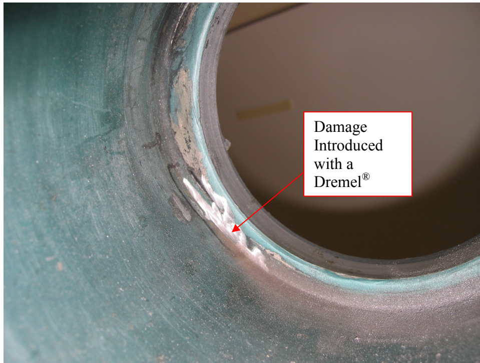
Figure 4.11. Damage introduced to structure
