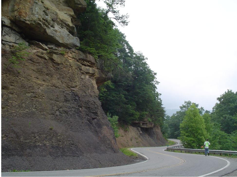
Figure B.5- Example slope in Campbell County (RHRS 355 additive; 395 multiplicative)
