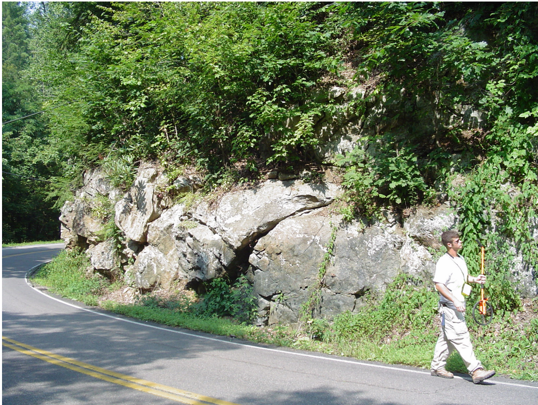
Figure B.6- Example slope in Unicoi County (RHRS 368 additive; 301 multiplicative)
