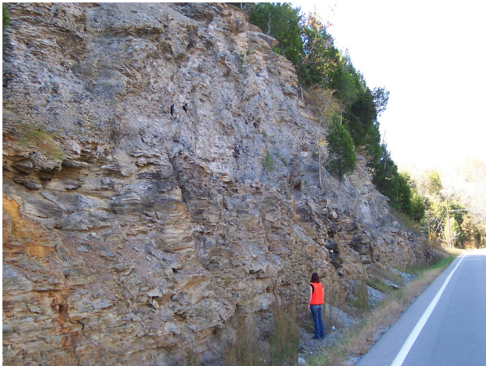
Figure B.8- Example slope in Cheatham County (RHRS 243 additive; 173 multiplicative)
