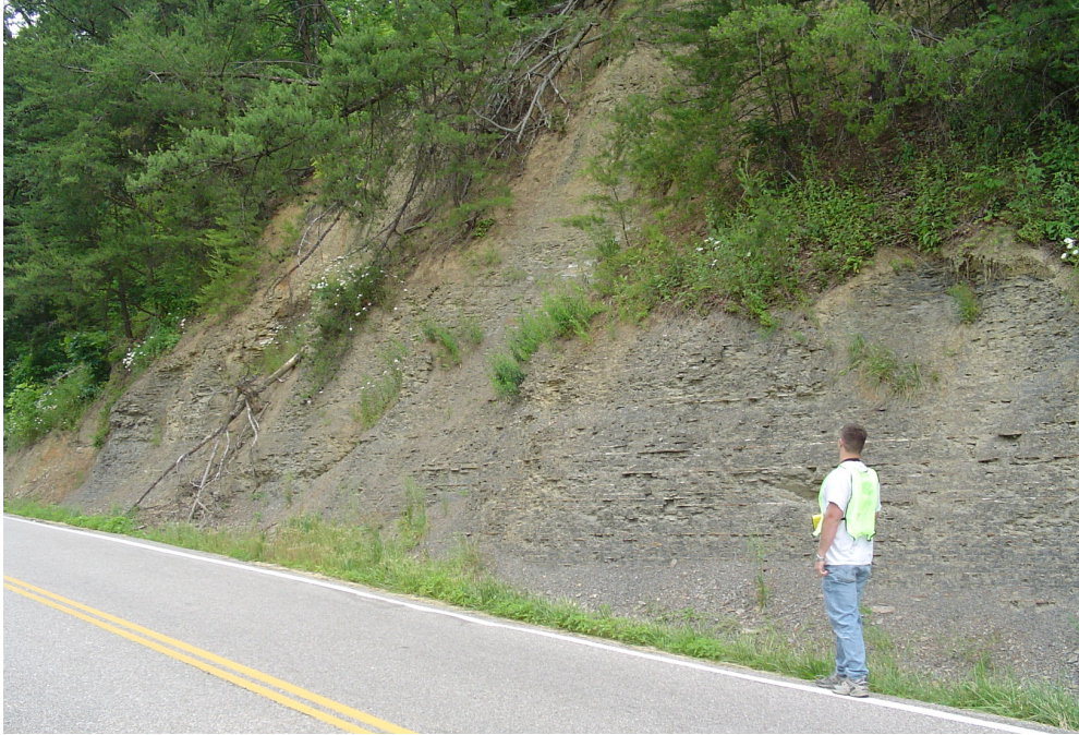
Figure B.4- Example slope in Campbell County (RHRS 228 additive; 152 multiplicative)
