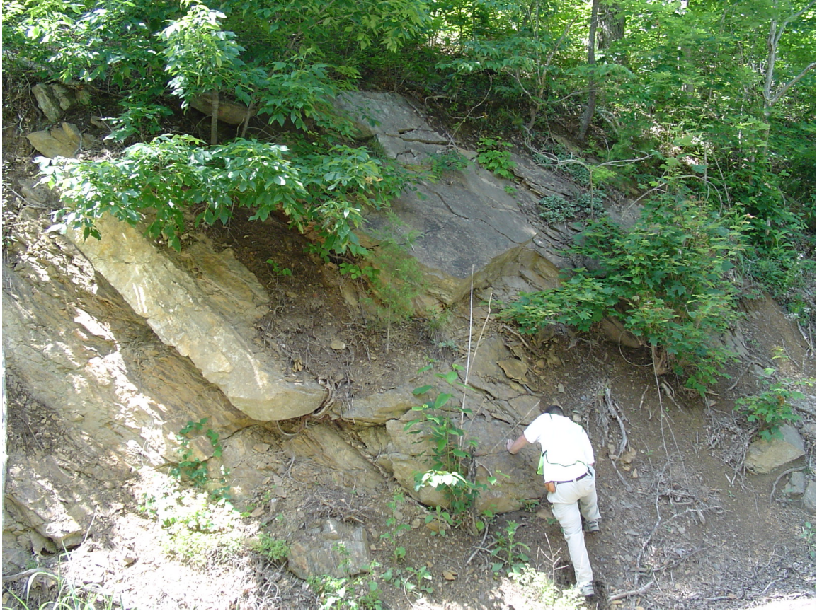
Figure B.7- Example slope in Hancock County (RHRS 242 additive; 246 multiplicative)
