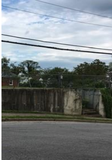
Figure 11. First Baptist Church Steps.
