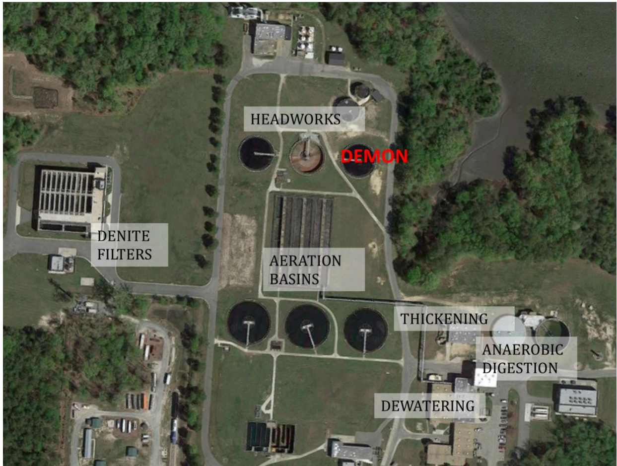
Figure 2: An aerial photo the Hampton Roads Sanitation District's York River Wastewater Treatment Plant with process annotations.
