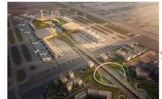
New Mumbai Airport
