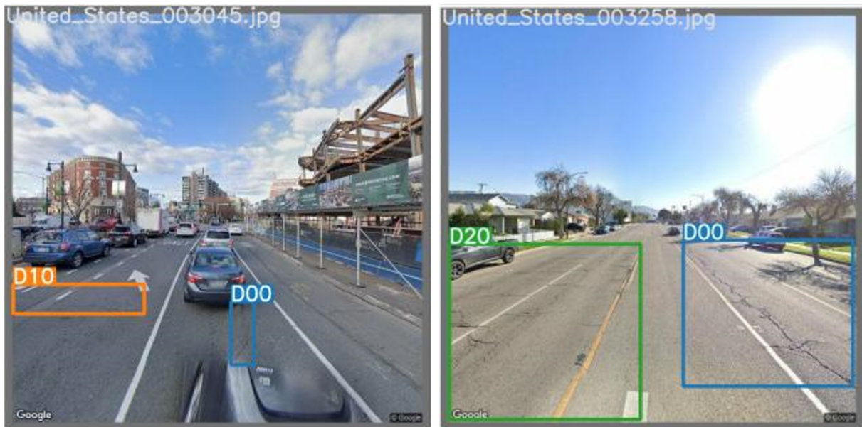
Figure 2.10: The images showcase two Google Street View (GSV) images. Each image was evaluated by a trained YOLOv7 model. The predictions are tagged by a category. The labels displayed D00, D10, and D20 are respectively longitudinal, transverse, and alligator cracks.
