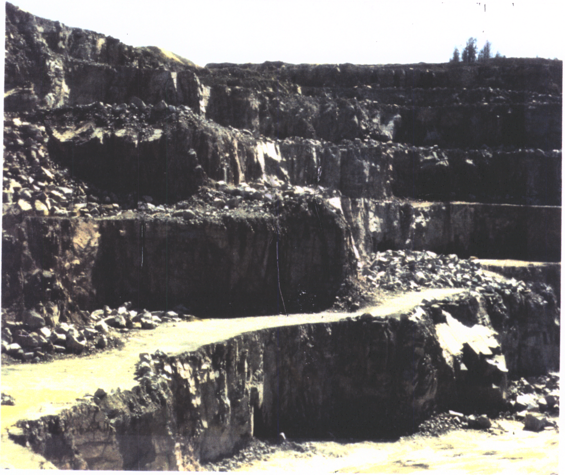
Plate 2.5 - Unstable Slope in Active Producing Area
