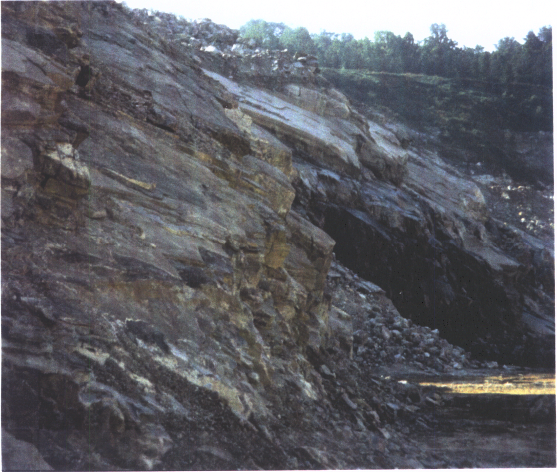
Plate 2.3 - Plane Failure
