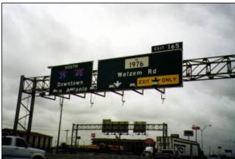
Figure 4.7 – Vertical Mounting Configuration for Southbound Coverage of I-35 at AVI Site 45
