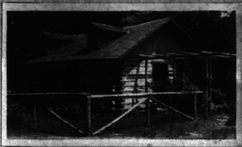
SHOWING OUTSIDE OF COMMUNITY HOUSE
