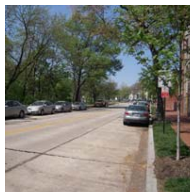
2 | P Street Bridge looking west
