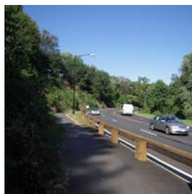
1 | Rock Creek Parkway
