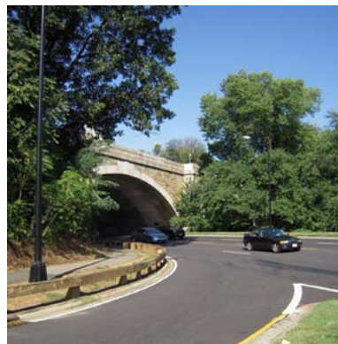
3 | P Street Bridge over Parkway
