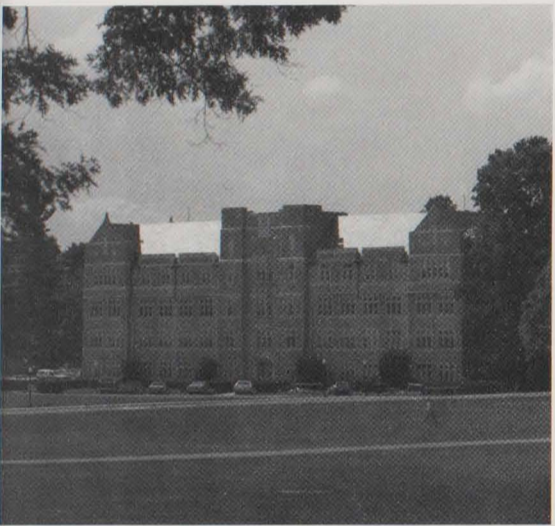
144. Davidson Hall, constructed 1938
