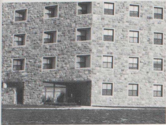
78. Solar responsive enclosure
