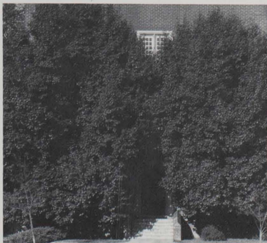
149. Plant material hazard
