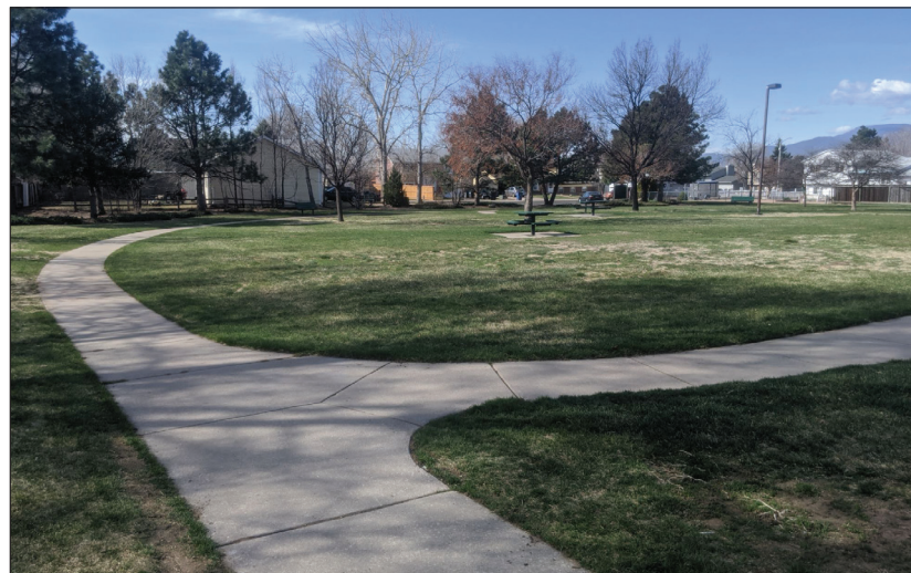
A 6' paved sidewalk runs throughout the main area of the site and is designed for universal accessibility. It could potentially be made of permeable asphalt.
