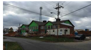
E - Entrance at East Main and Longview Drive
