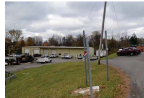
B - Entrance to existing City Garage
