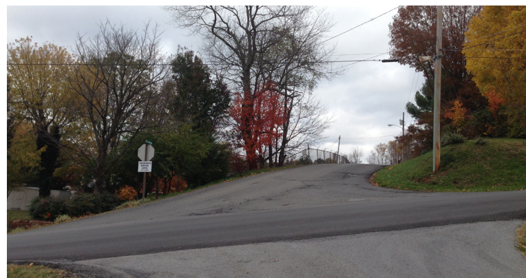
C - Entrance to the Municipal Garage Site from Lincoln Avenue
