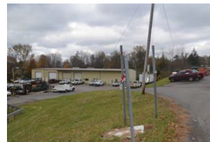
B - Entrance to existing City Garage
