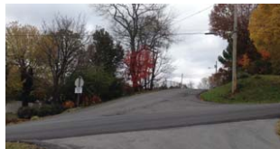
C - Intersection at Lincoln Avenue
