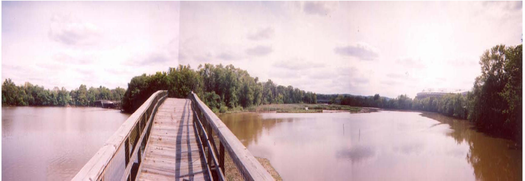
Figure 4.11 Foot bridge to Heritage Island.
