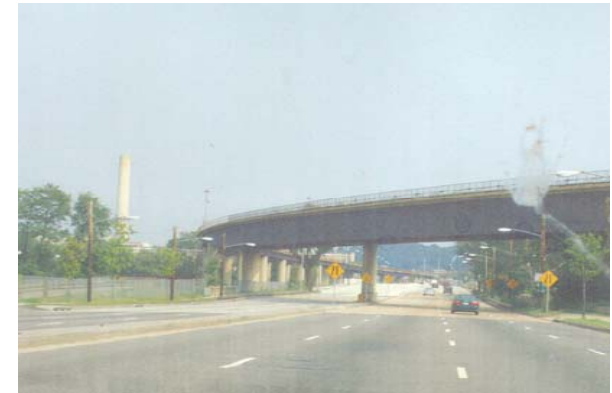
Figure 4.12 Benning Road looking east.
