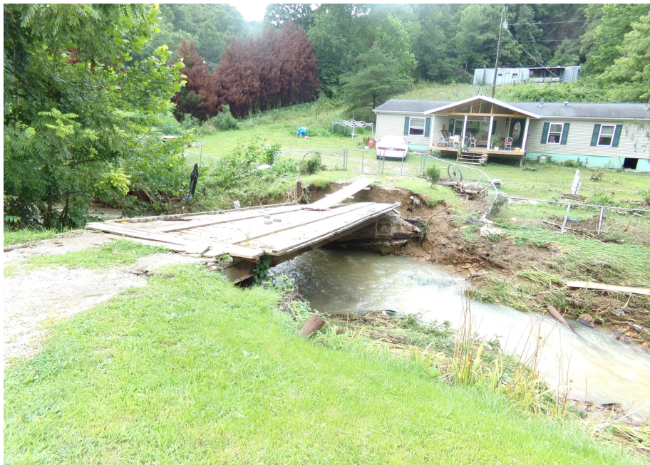
Figure 1: Private Bridge Example ( Bridge Program, n.d. )
