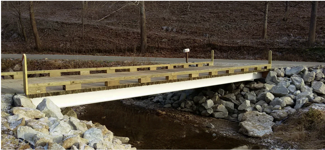
Figure 2: Private Residential Bridge After Bridge Home Program Replacement (Courtesy of WV VOAD)
