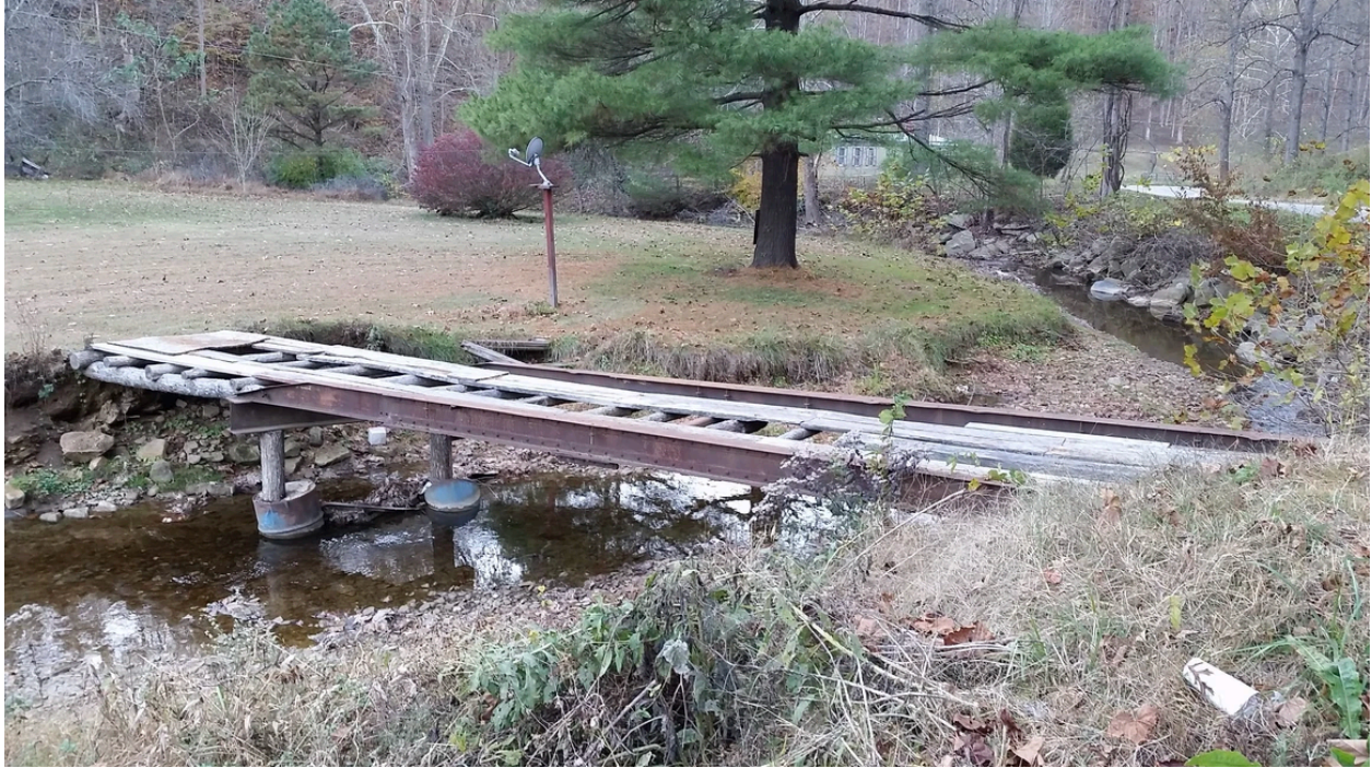
Figure 1: Poorly Designed Private Residential Bridge Before Bridge Home Program Replacement (Courtesy of WV VOAD)
