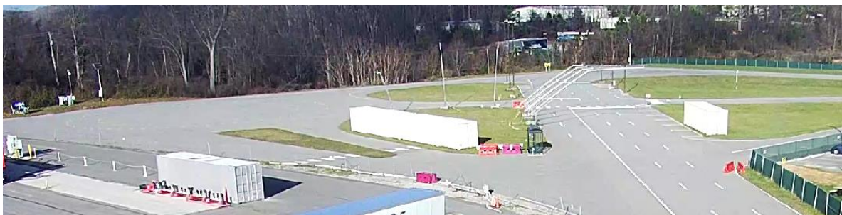
Figure 19. Top view of the Virginia Smart Roads Surface Street Expansion (SSE). Features include a large intersection, roundabout, and different lane configurations.
