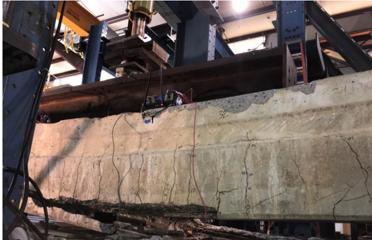
Figure 1.3. Flexural failure of prestressed concrete bridge girder [test conducted by Alfaiakawi et al. (2020) ].
