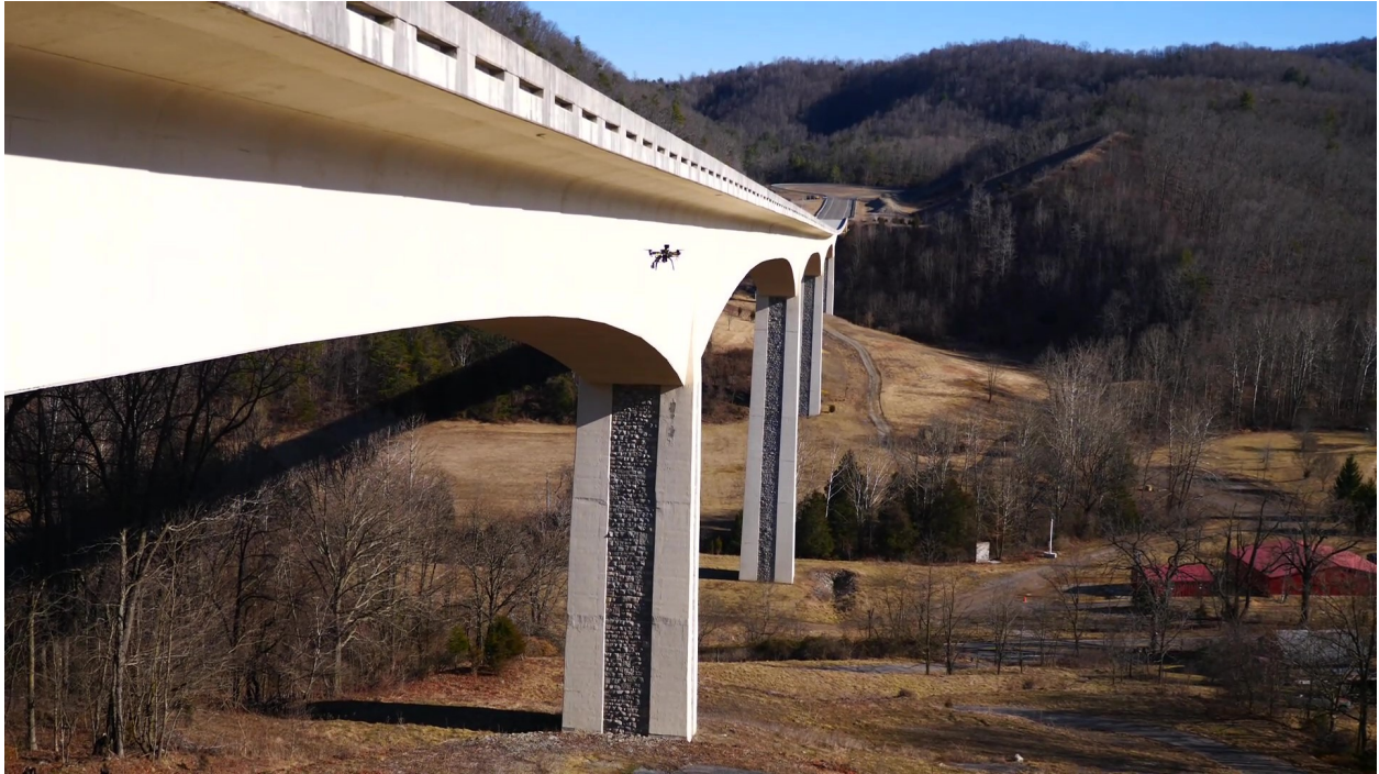
Figure 4.9: Experiment at the VTTI Smart Road Bridge.
