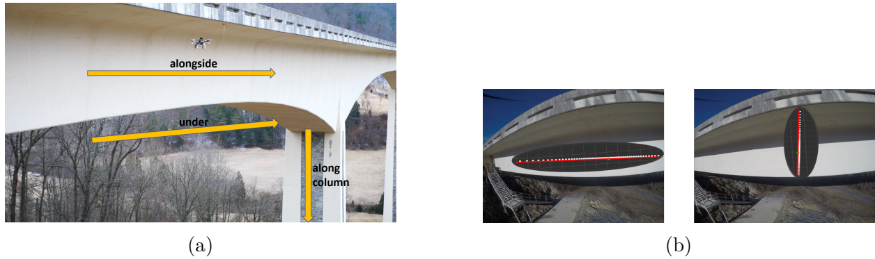
Figure 4.4: (a) Illustration of some useful navigation routines. (b) White dots: LiDAR data; Red line: best fit using Hough Transform.
