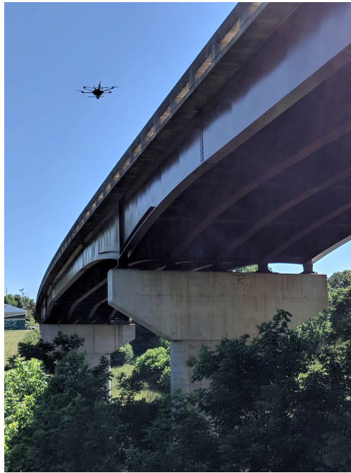
Figure 1.3: UAV conducting 3D visual inspection of a bridge.
