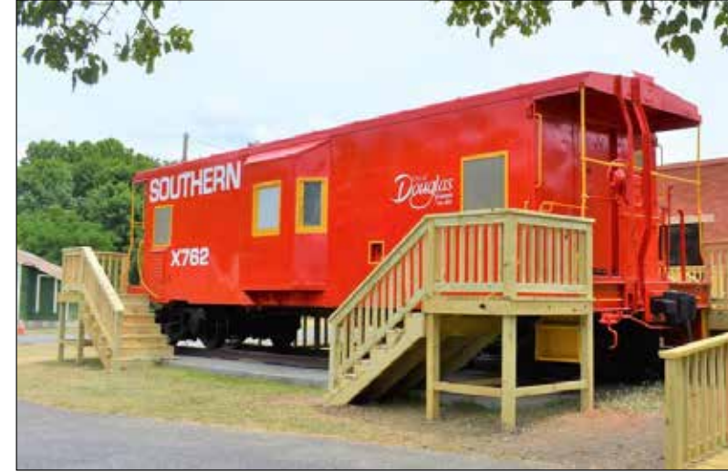
The renovated caboose includes a proposed staircase to make it easier to access the inside of the structure.
