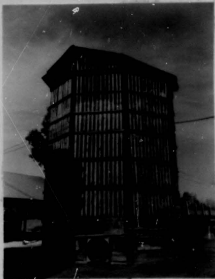
The Iowa Haykeeper - latest development for efficient storing, drying, and feeding chopped hay. Cost, approximately $1,000, capacity 50 tons hay.
