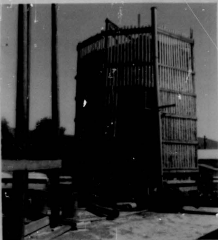
Structure for storing, drying and self-feeding chopped hay. Portable crop dryer (left) was used to dry the hay.
