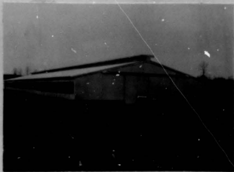
A 40 foot wide pole type poultry laying house, VPI Plan F-1.18A. Aluminum siding and roof, insulated roof and side walls, double layer clear plastic on windows, natural ventilation.
