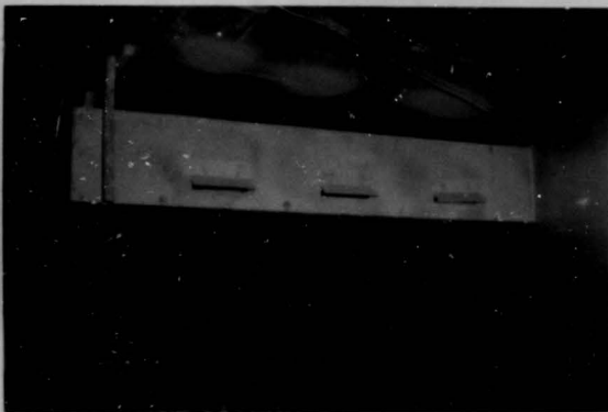
A pressurized poultry house ventilating system. Electric fans provide positive control of ventilation.
