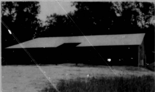
Building for market hog feeding operation on the J. J. Lilley farm.
