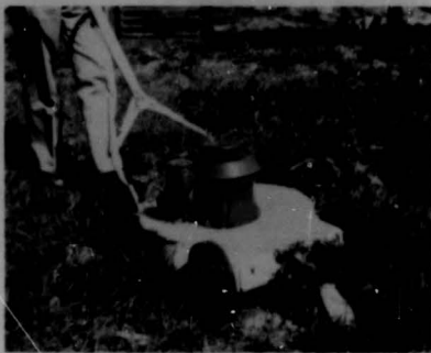
Note rock hidden by weed from operator's view.
