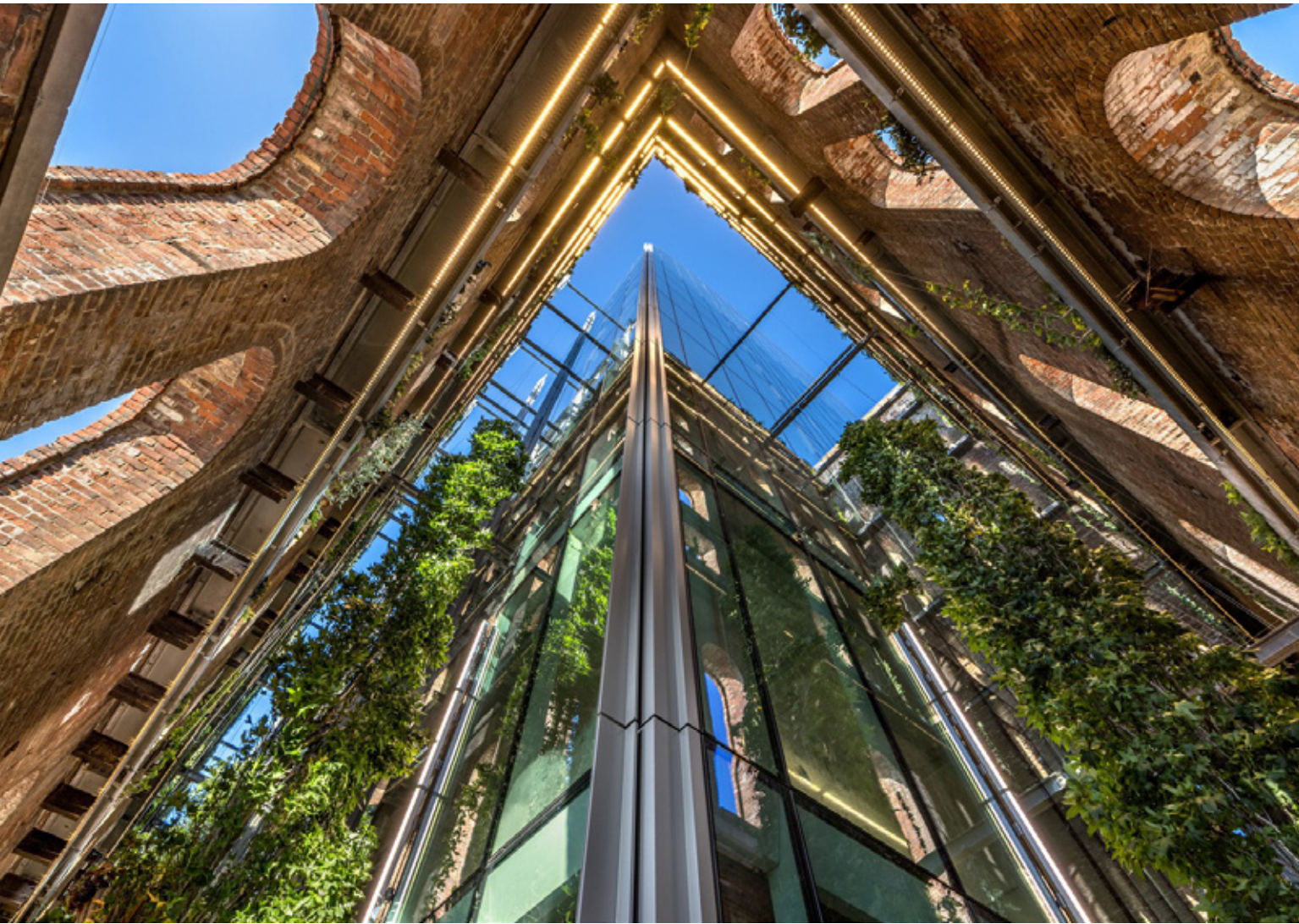
Figure 20: Looking up at the void space between existing facade and new structure/ Sources: https://www.archdaily.com/1007905/domino-sugar-refinery-pau
