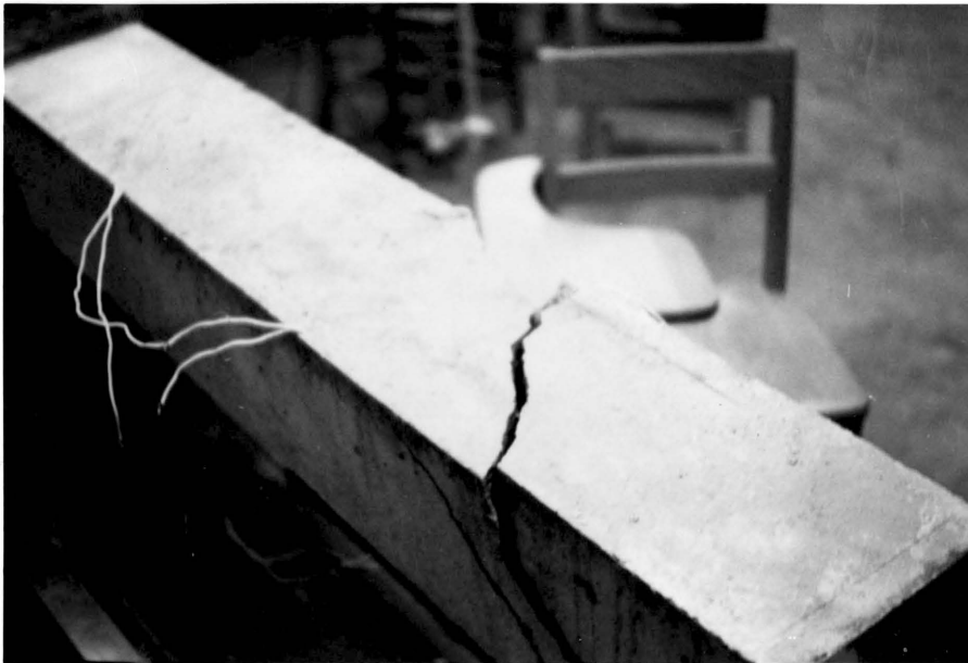
Figure 3-45 Failure Cracks, Beam 2-4
