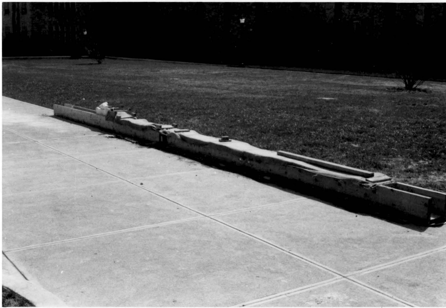
Figure 3-1 Beams Curing in the Forms
