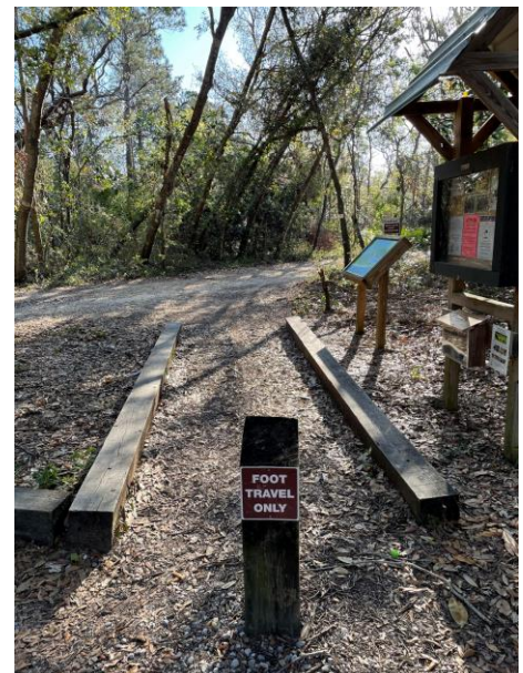
This bollard reduces the trail width significantly enough that it prevents wheelchair and scooter users from accessing it. Photo: Freya McGregor.
