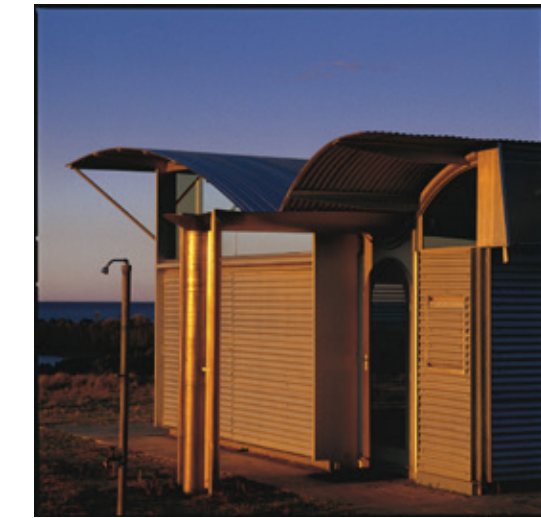
figure 55. Gutter and downspout
