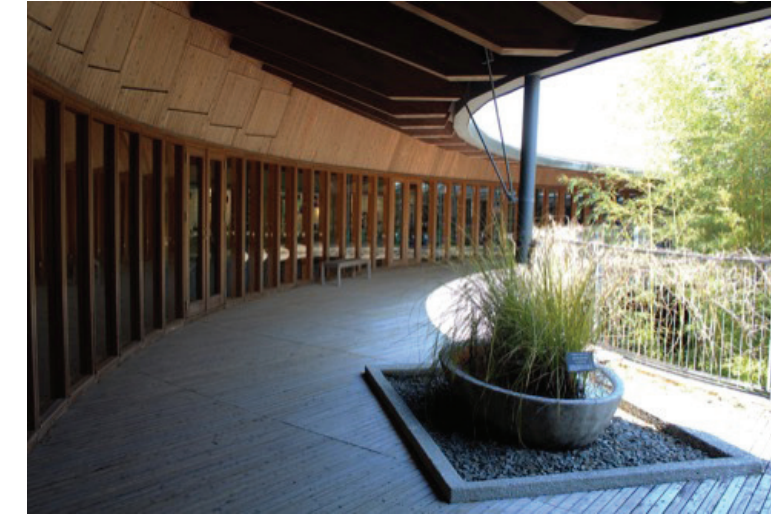
figure 53. Gutter and downspout
