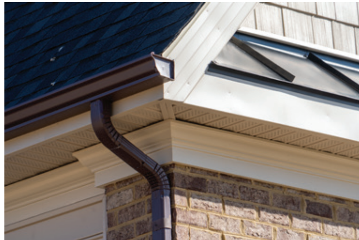
figure 44. Gutter and downspout
