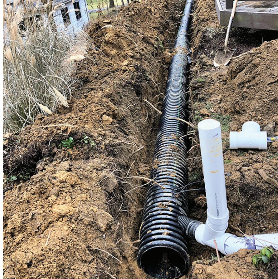
figure 39. French drain system
