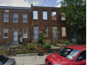
figure 69. Photo of site 3-2
