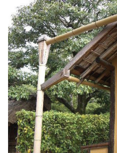
figure 46. Gutter and downspout
