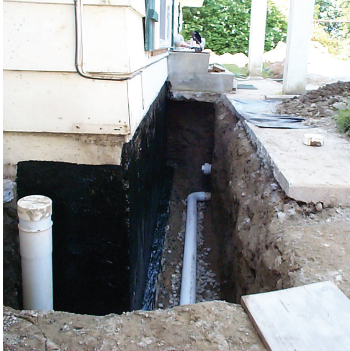
figure 41. Footing drain System
