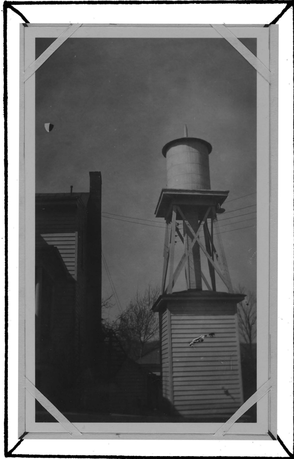
Water tank and spring house
