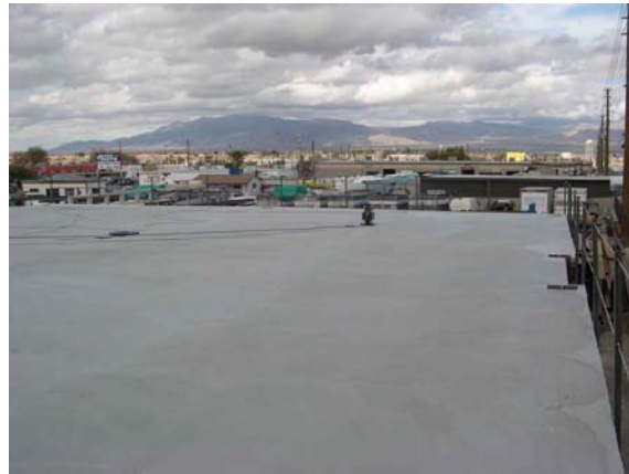
Figure 4.13: Long Span Composite Slab Mockup Picture
