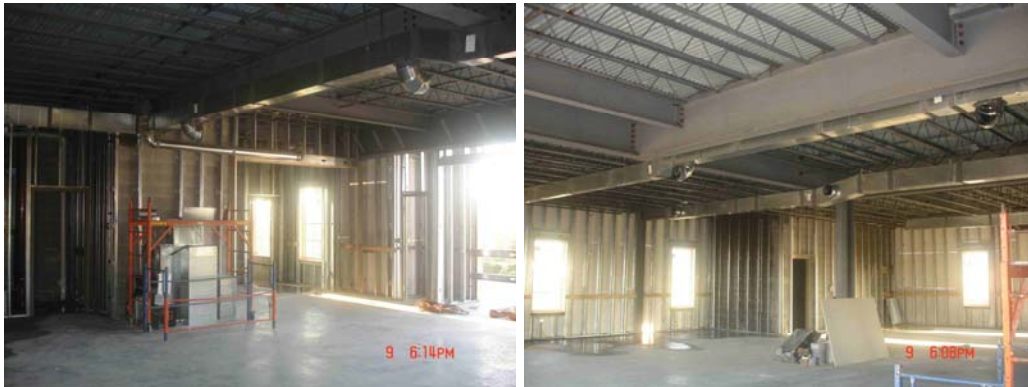
Figure 4.75: First Bank & Trust Building Slab Underside
