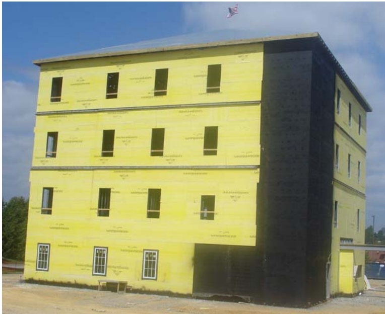
Figure 4.73: First Bank & Trust Building (During Vibration Tests)
