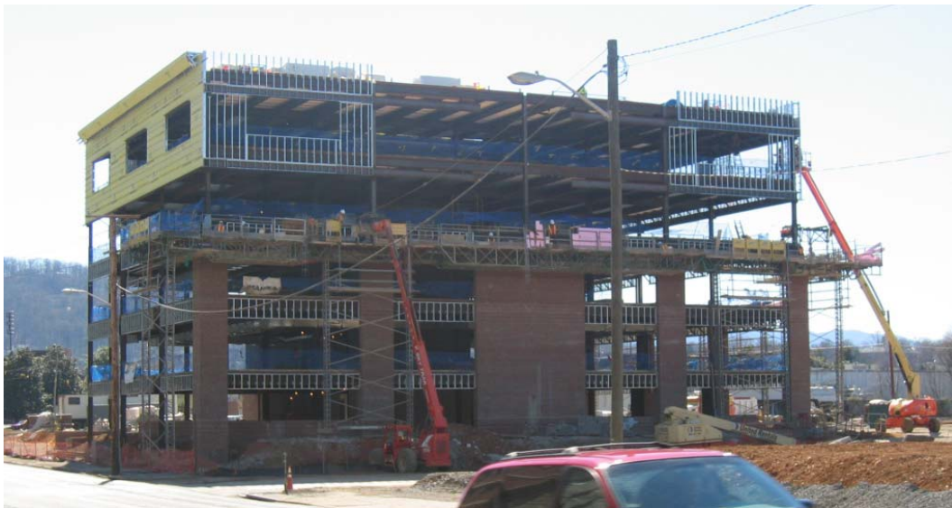
Figure 4.52: Riverside MOB (During Vibration Tests)
