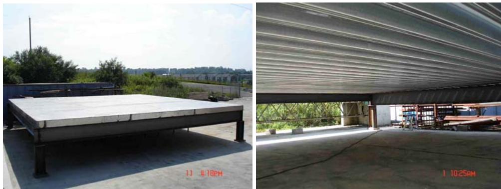
Figure 4.1: Long Span Composite Slab Specimen Pictures
