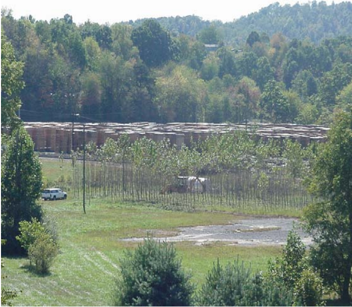
Wide Angle View of Oneida Poplar Tree Phytoremediation System
