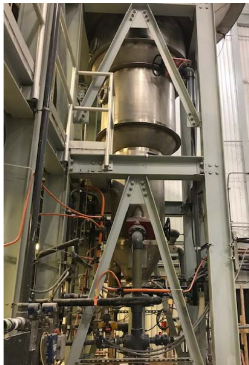
Figure 58: Upper Wet Harvest Leg of Pilot Reactor (R3)
