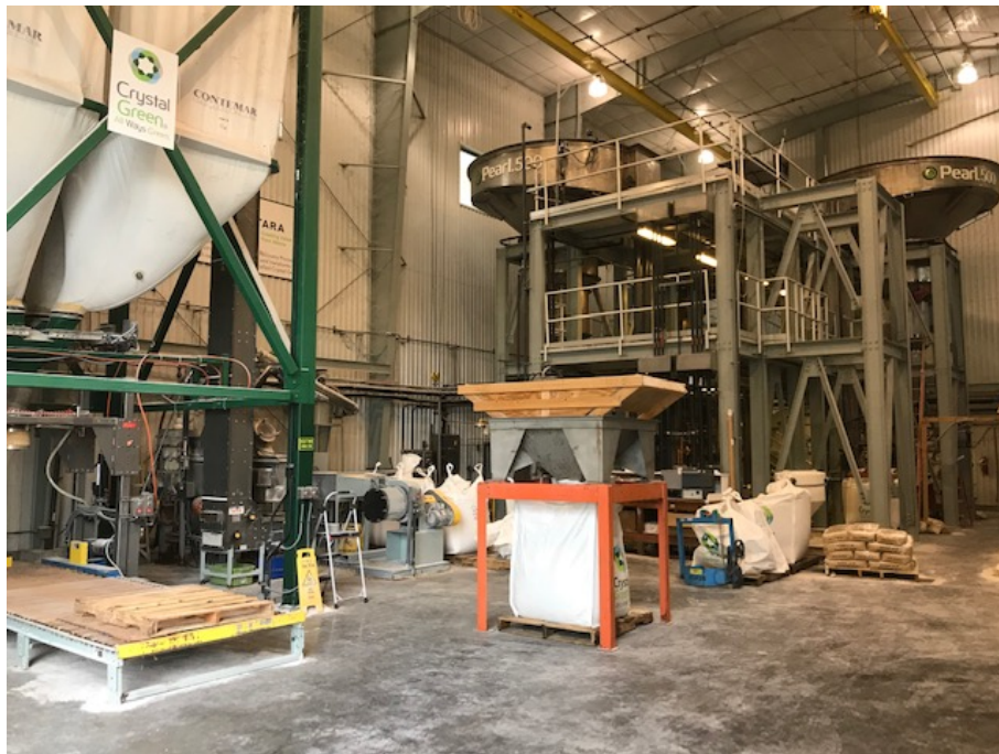
Figure 6: HRSD Nansmond Treatment Plant Struvite Recovery Facility (SRF)
