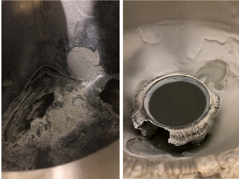
Figure 34: a. Scaling of Lower Portion of Reactor 1 after 3 Months of Operation (July 2019); b. Scaling of Lower Portion of Reactor 1 after 9 Months of Operation (September 2020)
