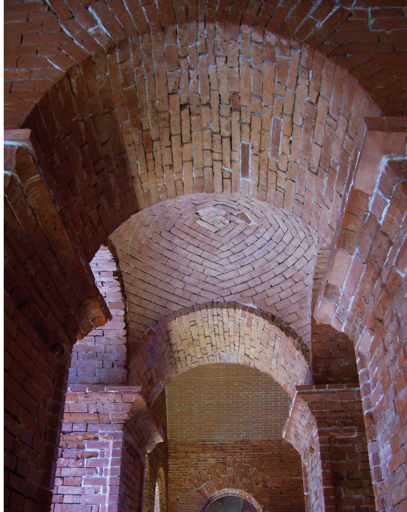
Brick Vaults, Munich, Germany
