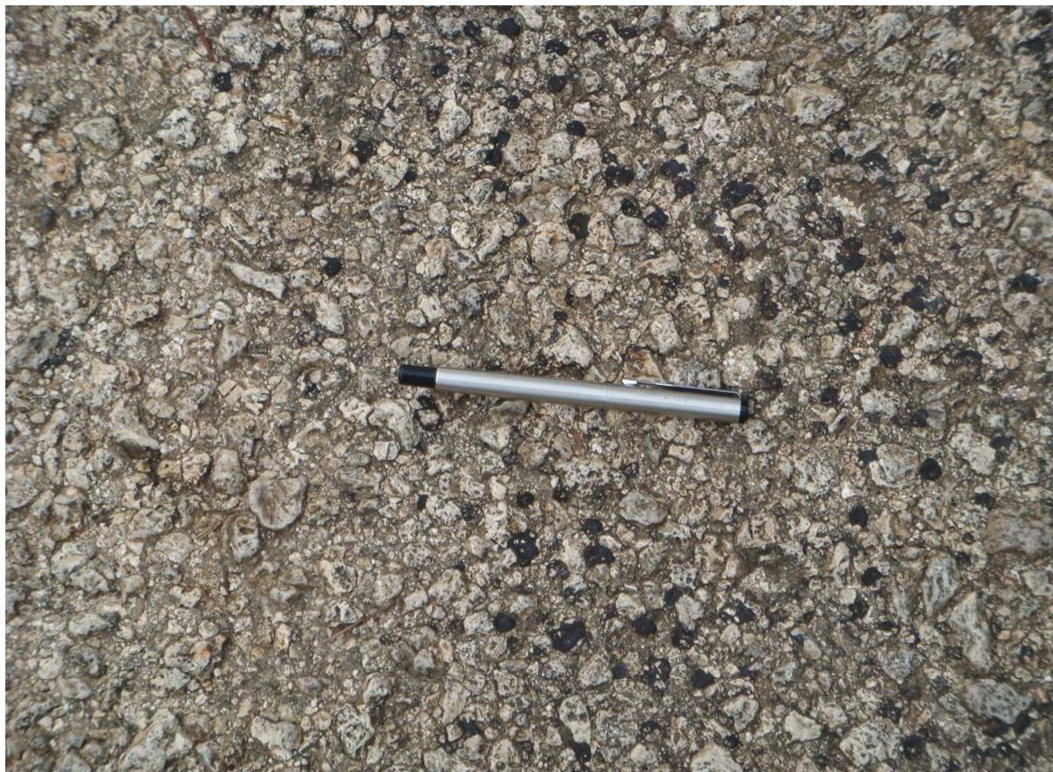
FIGURE 2 Close-up of Otta seal surfacing on Folaha Road constructed in August 2012.
