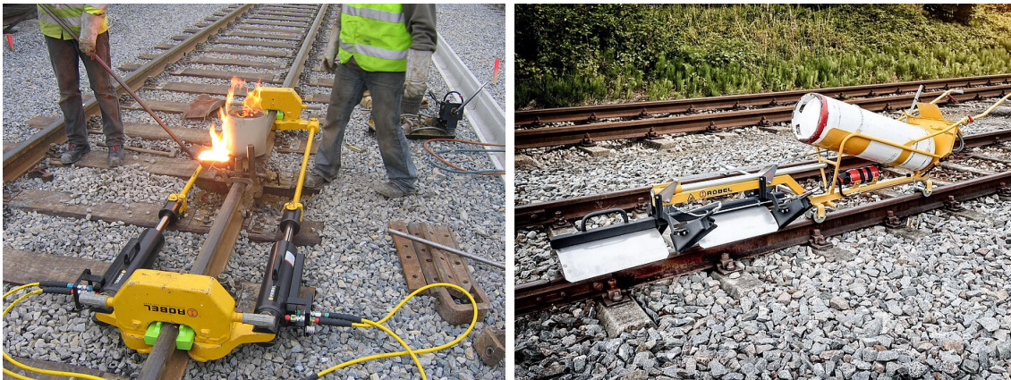
(a) A hydraulic rail tensioner.
