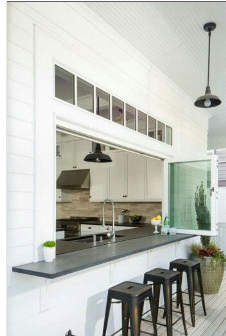
An opening near the reception area allows increasing visual access and interactions with visitors throughout the building. A transom is added to match the existing transoms found above other doors.
