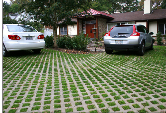
Permeable pavers offer an environmentally-friendly surface alternative for low-traffic vehicle areas. Permeable paving minimizes stormwater run off and reduces pollutant migration.
