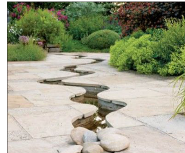
A small channel diverts collected stormwater into a rain garden, encouraging curiosity about local geology and hydrology.
