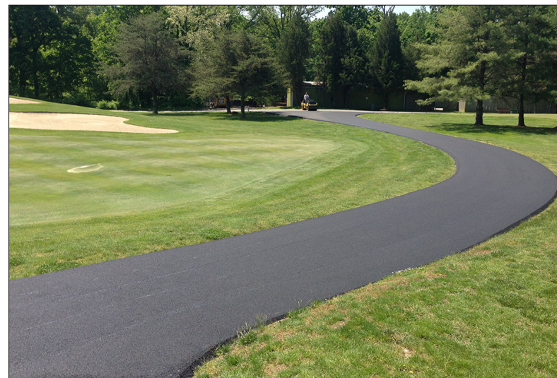
Asphalt is a cost effective and durable surface option for many of the walking trails around the site that is universally accessible.
