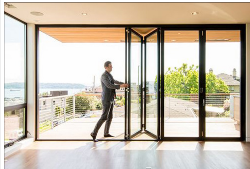
A folding glass door added to the multi-purpose community building creates a seamless transition between interior to exterior spaces.
