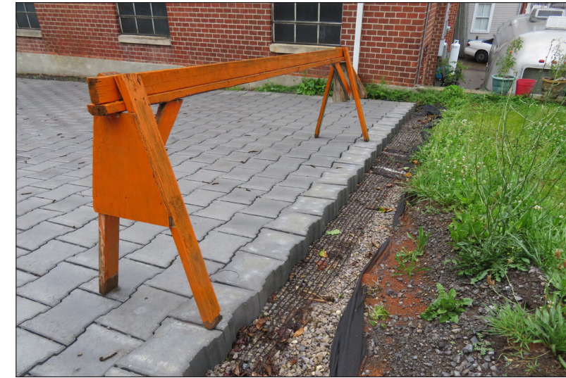
Permeable paving in the parking lot uses an interlocking system of concrete blocks that is durable and absorbs stormwater runoff.
