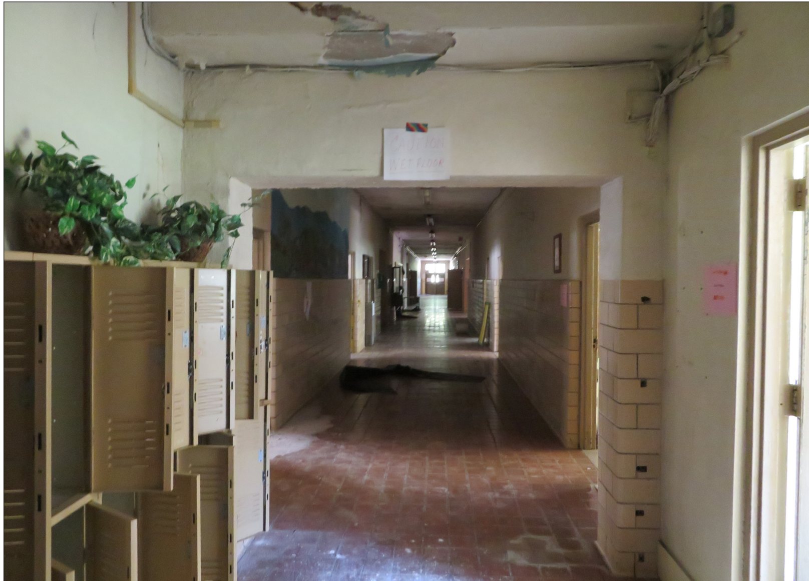
The view from the stone building into the brick addition.
