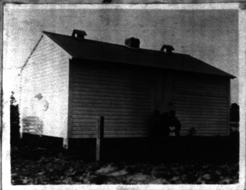
No. 4 shows Dr. Griffin newly constructed Potato curing house.
