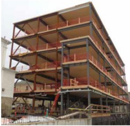
(a) Structure during construction
