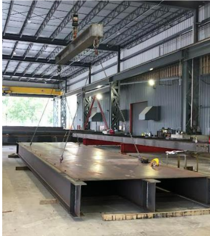
Figure 6-12. Lifting of whole module for placing on truck
