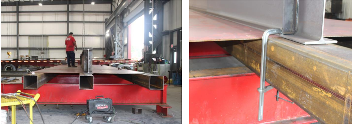
Figure 6-5. Placing of center beam
